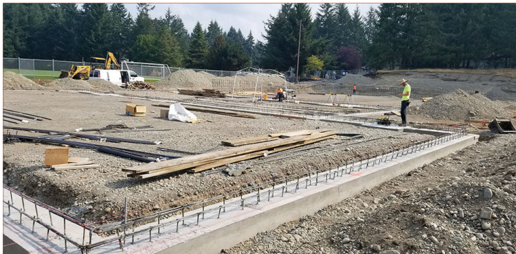
River Ridge High School Auxiliary Gym under construction, August 2018
